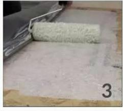
Apply adhesive to deck and roll the Membrane back out whilst the adhesive is still wet.
