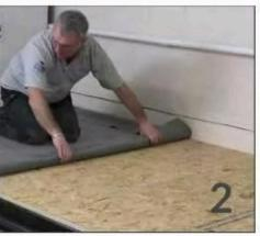
Lay out membrane and allow to relax for 30 mins. Then roll the rubber to centre point starting from one edge.
