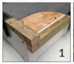
Ensure battens have been installed around the roof perimeter and along the face of gutter edge.
