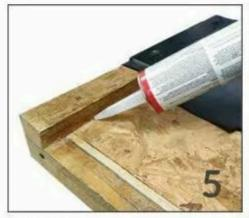
Apply supplied mastic to perimeter of roof before folding rubber over the edges.
