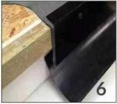
Cut to size metal trim and Face fix along the Gutter edge (Use supplied joiners if required).
