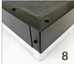
Apply metal corner pieces and complete installation by cutting off any access membrane.
