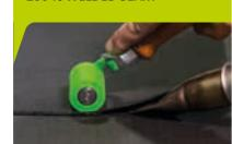
The bitumen layer on the underside of the membranes melts when welded with hot air and the overlapping RESITRIX® membranes weld to each other. The entire process happens through temperature, pressure and time. Heat melts the polymer-modified bitumen of the upper layer. Pressure pushes the two compatible membrane layers together. What emerges at the end is the weld bead – your visible
