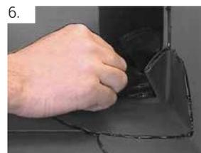
Remove the protective film in the inverted pleat area and weld it with hot air. Fix the inverted pleat to the upstand using migrated bitumen from an off-cut.
